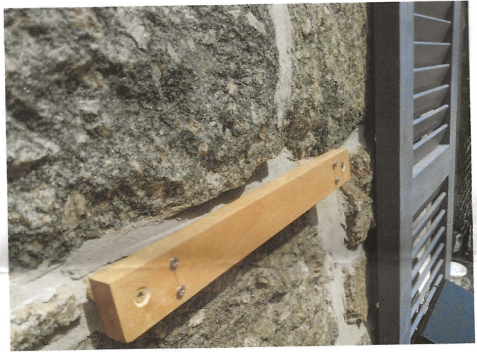
Mounting board attached using anchors
