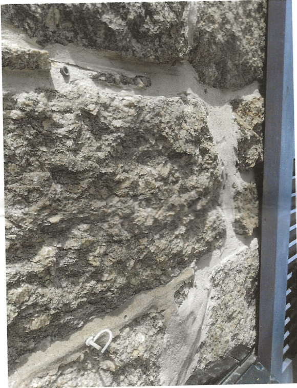
Existing anchors and cable clip on wall
