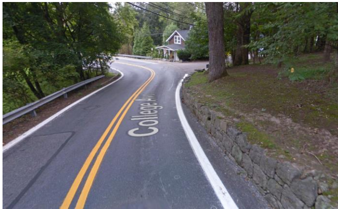
Figure 17 - Original location of wall
