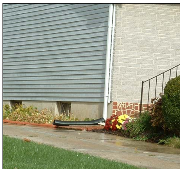
Figure 1: Downspout Intentionally Bypassing Landscaped Area and Draining onto Driveway
