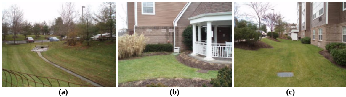
Figure 3.12. (a) Concrete channel in stormwater pond could be retrofit to provide water quality treatment at NSA_21; and (b & c) Rain garden or bioretention potential at NSA_21.
