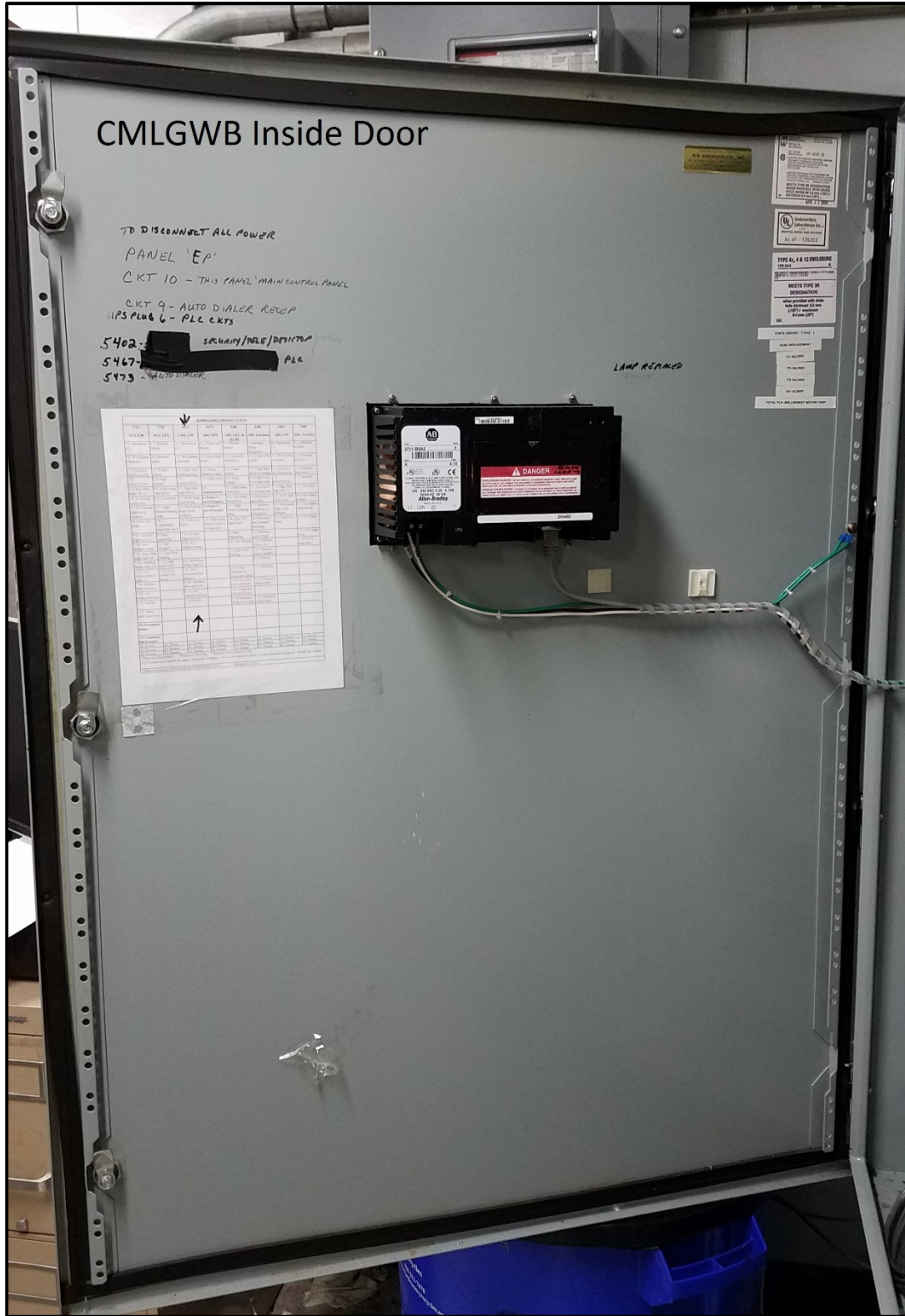
Figure 2: Carrs Mill Landfill GWB Enclosure Door Inside
