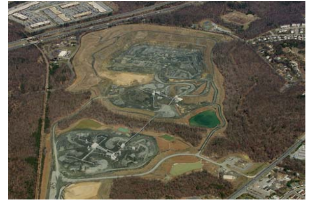
Post-reclamation concepts for the Chase Quarry in Jessup include mixed-use residential and employment development with community amenity space.
